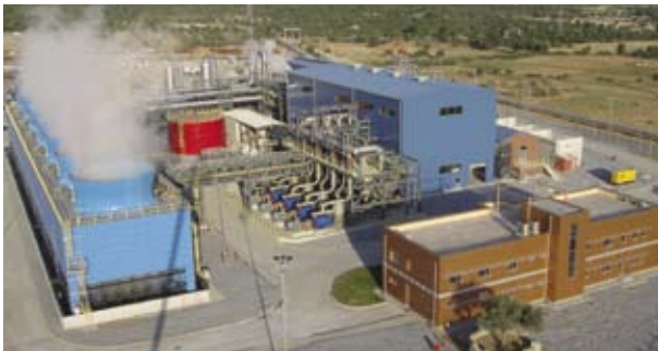
High Potential: Local sponsor Germacik's 47.4 megawatt facility is the largest geothermal plant to date in Turkey.
